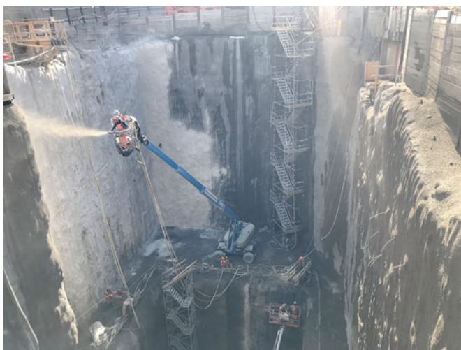
Figure 6 Excavation of Entrance Shaft
